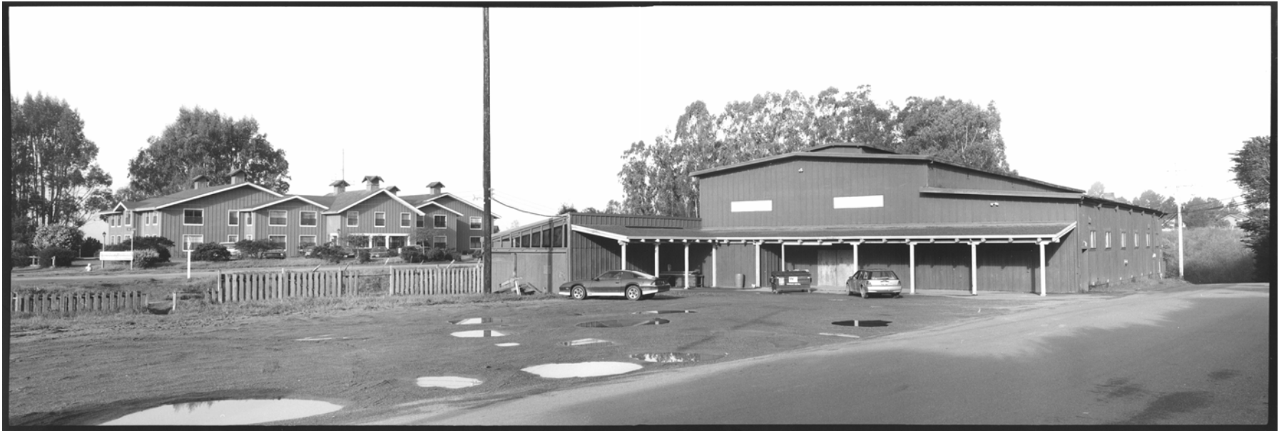
The old railroad barn on Mesa Road; across A street, Walnut Place
