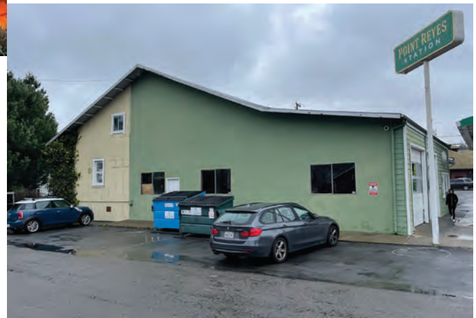
West end of building, showing stuccoed portion of exterior wall, January 21, 2024.
