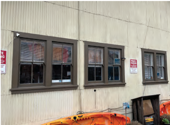
Historic window fabric and placement, January 21, 2024.
