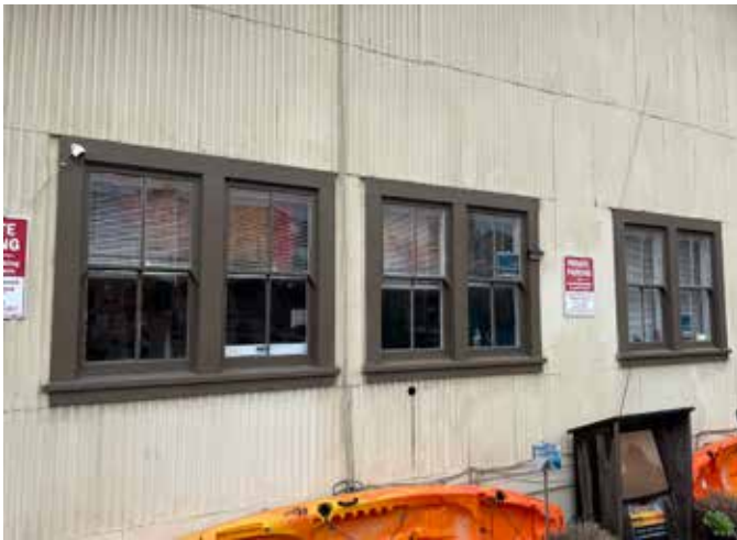
Historic window fabric and placement, January 21, 2024.
